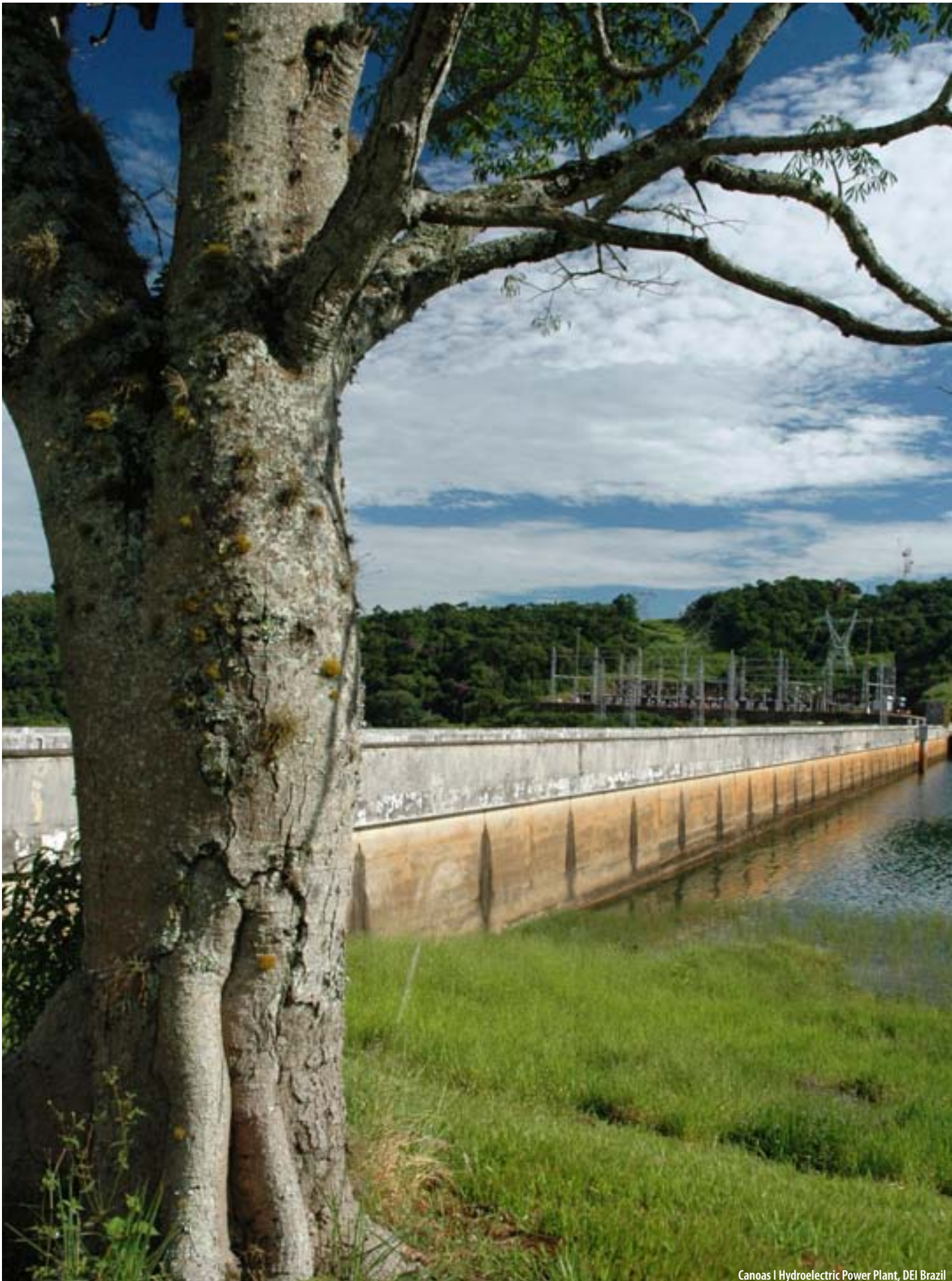
Canoas I Hydroelectric Power Plant, DEI Brazil
