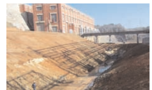
Excavation at the bottom of Wateree Dam
