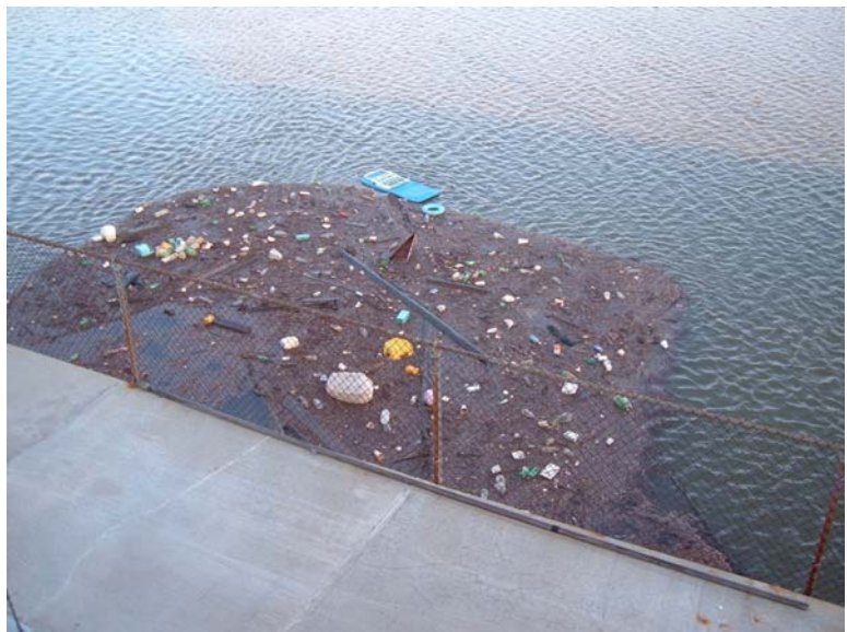
Trash collects gradually during normal operation.
