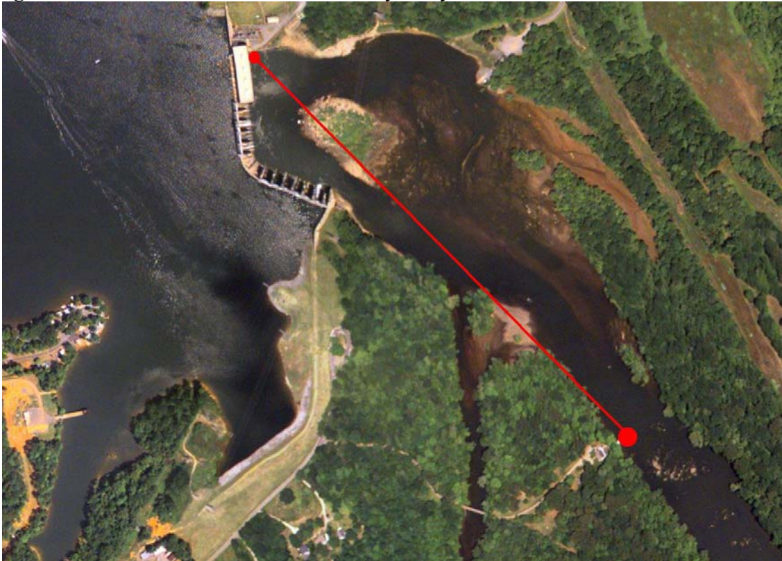
Figure 2. Recommended Location of the Wylie Hydro Permanent Monitor
