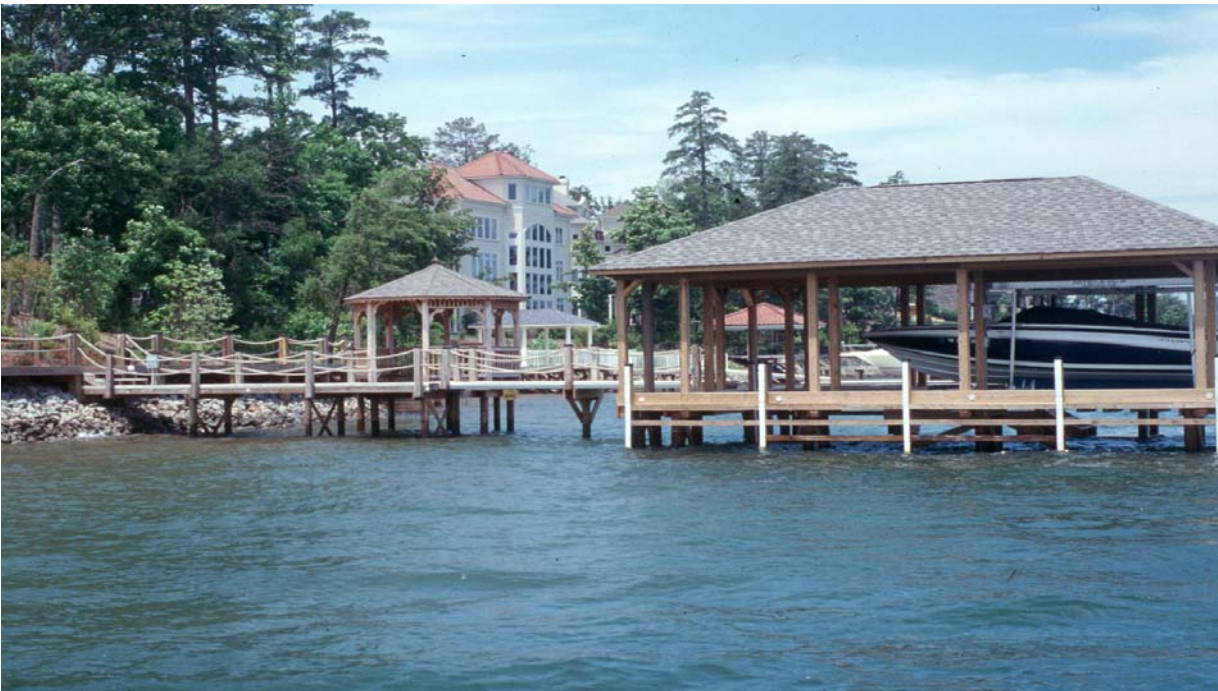
Riprap/Piers--Shorelines with riprap or piers that intrude into the reservoir.
