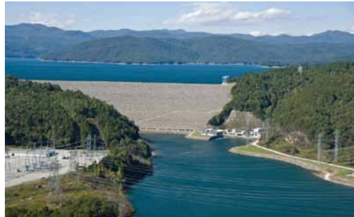
Jocassee Hydro Station
