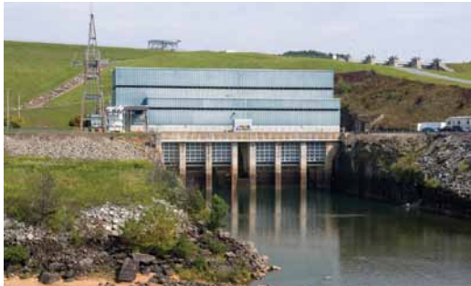
Keowee Hydro Station
